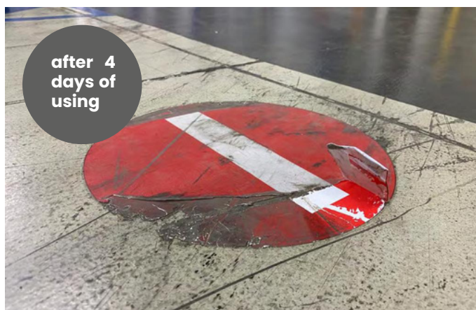
polyester laminated tape on the highly frequented place
